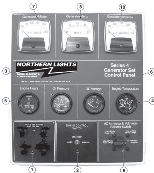
Figure 8: Series 4 B Generator Control Panel
