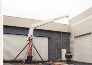
Cranes are proof tested to 110% of capacity
